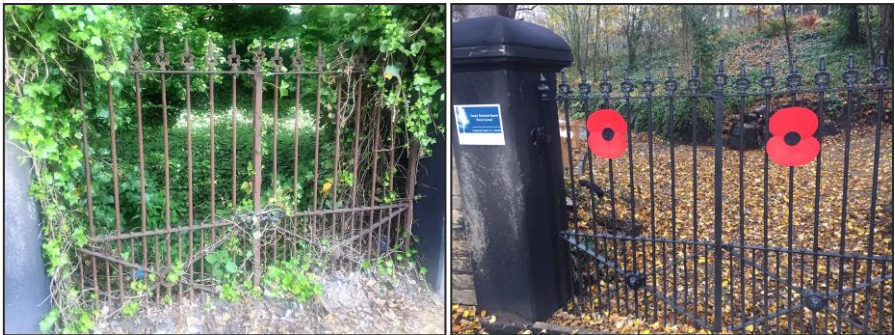
Before and after work on the entrance gates Photographs courtesy of John Barker
