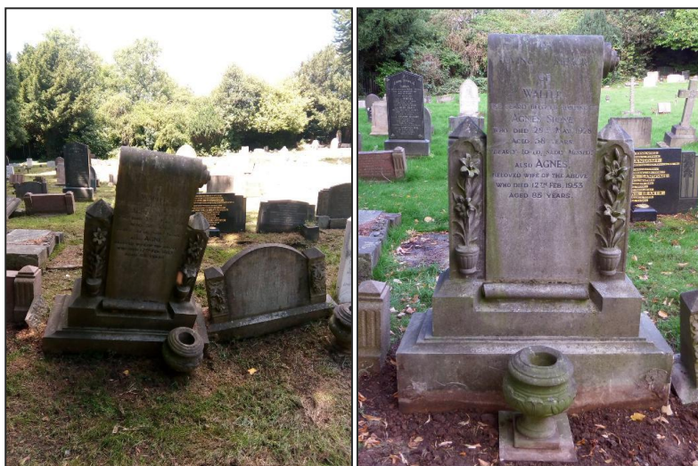
The Walter Stone memorial before (left) and after repair (right) Photographs courtesy of Dorothy Marshall
